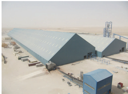
Gulf Cement Company, Umm Bab, Qatar
