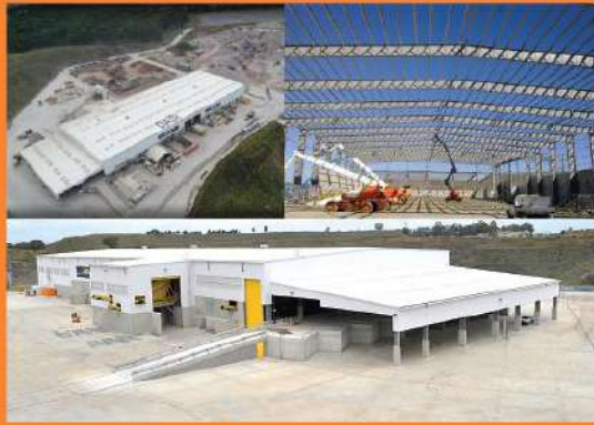
Industrial Bingo Eastern Creek Recycling Factory
