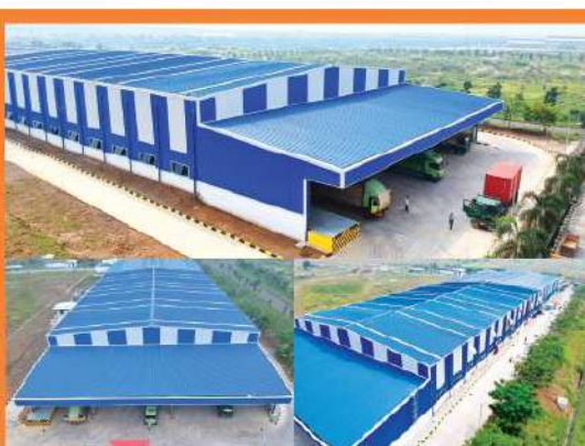
Industrial Asian Paint Karawang Factory
